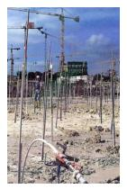
SiliBond®SI 711 replaces, under ecological and technical advantages, in these applications the classical soluble sodium silicate injection. It is almost completely free of ecologically harmful substances and largely pH-neutral. The water glasses typical, high alkalinity is completely eliminated in this injection material.
