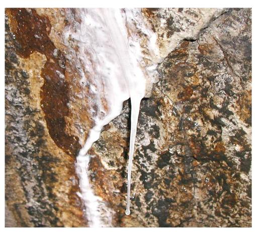
Application: Sealing a crack in a tunnel with high water flow with Hydro-Bloc®575 Integral.
