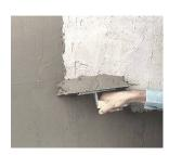
Silex®961 can be applied by hand or sprayed with the usual tools. When applying by hand, it is advisable first to submit a thin layer under strong pressure ("crunching") and then rework "fresh in fresh".
