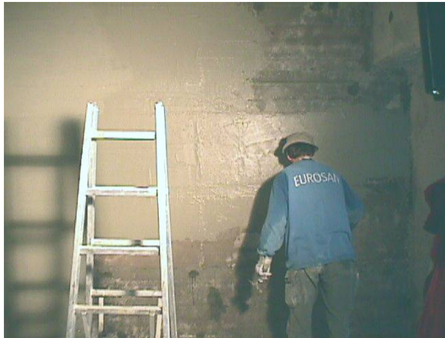
Restoration and waterproofing work on extensive wet, salt-loaded concrete walls of an underground car park with Cembond®M-945.
