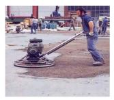
HydroBloc<sup>®</sup>EP Curing 904 can be worked into concrete while smoothing, or after 24 hours the latest by rolling or spraying
