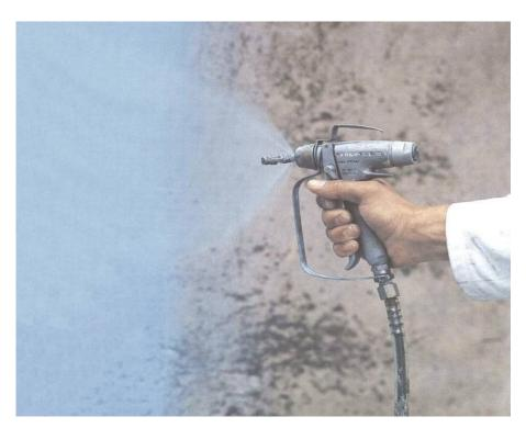
The underground should be dry, clean and free from all separating substances. Pinholes, air porous and crack more than 0,1 mm width as well as other damages in concrete surfaces need special treatments e.g. with UP®-Steinspachtel 1013 which is highly recommended for this application.
