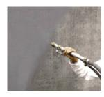
Silox®860 D is applied manually with the usual tools (spatula, trowel, wall scraperl, notched trowel) and can also be sprayed like thin layer plasters or sealing slurries with light spraying machines ( screw pumps ). Depending on the spraying pressure and the supporting air volume, more or less fine-rough structured, even surfaces are created.
