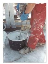
For mixing larger quantities and for highly filled mixtures, we recommend the use of compulsory mixers. For optimum mixing results with short mixing times, it is often advisable to charge the mixer with the liquid component already premixed from the master resin and hardener component.
