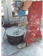
All substrates must be clean and load-bearing. Substances that have a separating effect must be removed without leaving any residue. To ensure adequate wetting of the substrate, the resin must be applied to glossy, wet substrates in such a way that the water film on the surface of the building material is displaced (**slurrying**). This is not possible by simple application with a squeegee or trowel.
