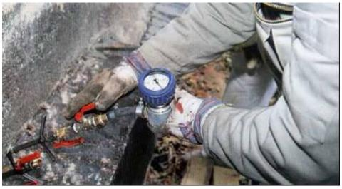
The classic pressure injection, via filler necks ("packers") into holes arranged in a grid
