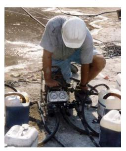
HydroBloc®Polygrout 650 mixed with water as a reactant, is injected into the areas affected by leaks by the usual methods using a high-pressure process. The rapid reaction between resin and water usually requires the use of injection pumps with suitable or adjustable mixing ratios for the two components, master resin and water. The mixing itself takes place directly at the injection point by bringing the two components together in a mixing tube, preferably with a static mixer as mixing element.
