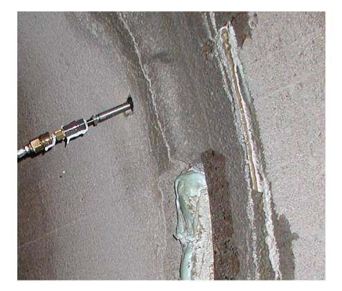
Sealing of movement joints in the pump channel of a sluice by filling the joint gap with HydroBloc<sup>®</sup>Rapid 570. Injection was performed at low pressure, from bottom to top. The packers were equipped with ball valves for control and to drain the water in the joint.
