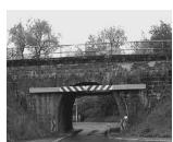
Waterproofing of a railway bridge: The completely saturated vault of compressed concrete and pre-masoned sandstone is now - after full-surface injection with HydroBloc® Polygel 530 - perfectly watertight again.
