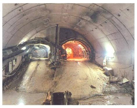
The line "METEOR" of the Metro in Paris. HydroBloc®Polygel 530 is certified from RATP the operating company for waterproofing work. It is also used for permanent repair work in the older parts of the transport network.
