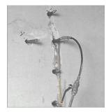
Regarding to the mixing ratio, HydroBloc®PU 500 can easily be used with all 2 component machines which can be adjusted to a mixing ratio of 1:1.
