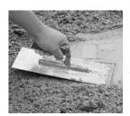
The ready mixed mortar will be applied with trowel on smaller areas or distributed with coating knife and smoothed or skimmed with a aluminium slat on devices. Additional compacting is not necessary. Devices made of polypropylene are suitable because the hardened mortar won't stick at this material.
