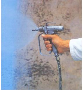
Silox<sup>®</sup>EPW 857 consists of 2 components. The mixing ratio is 29,94 : 5,74. It is possible to adjust the proper paint and spray viscosity with clean water.
